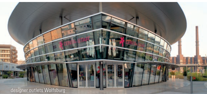
designer outlets Wolfsburg
